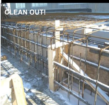
Make sure we cover the tops of forms for walls & footings at the end of the day to protect from weather.
